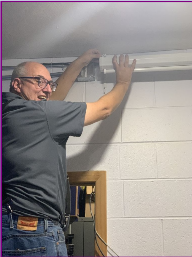
Installing projection screen
