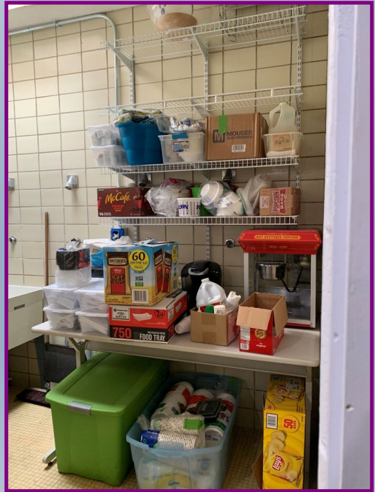
Kitchen shelving install
