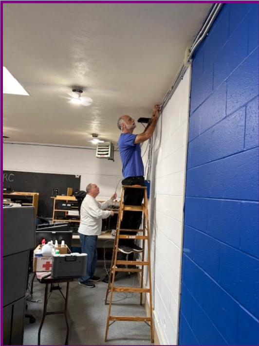
Ethernet and HDMI cabling install
